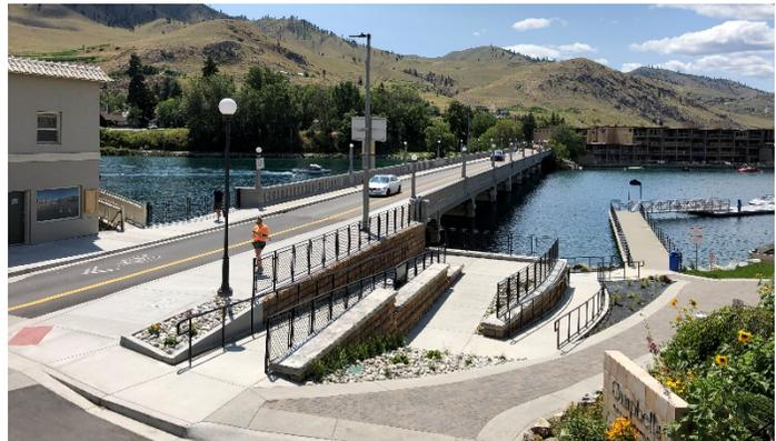
For more than a decade Chelan had been trying to figure out the best way to address Woodin Avenue Bridge safety issues, with its shifting and crumbling concrete, faulting electrical, and narrow sidewalks. Although structurally sound, renovations were sorely needed for this front door to downtown. The city had outgrown the narrow concrete bridge, originally built in 1927, and there was no longer enough room for all the pedestrians, bicyclists, and vehicle traffic.
